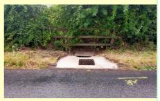
County Highways installed this gulley which connects to the existing pit which carries the water by pipe
