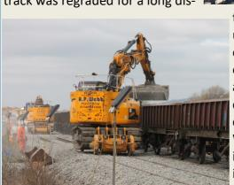
tance to make the change gradual. To be fair, it was a well oiled procedure removing the old track and ballast, relaying and regrading the new track including the replacement of the crossing in less than 48 hours. Weekend road closures are still in place to accommodate working elsewhere.
